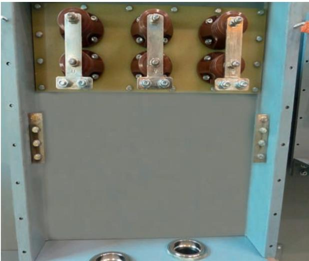
Example of a stator terminal box
